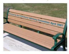
The bench slats are constructed from recycled plastic materials and backed by a 50 year warranty. The legs are made of coated aluminum. Regular maintenance will be completed on the legs, due to weathering.
